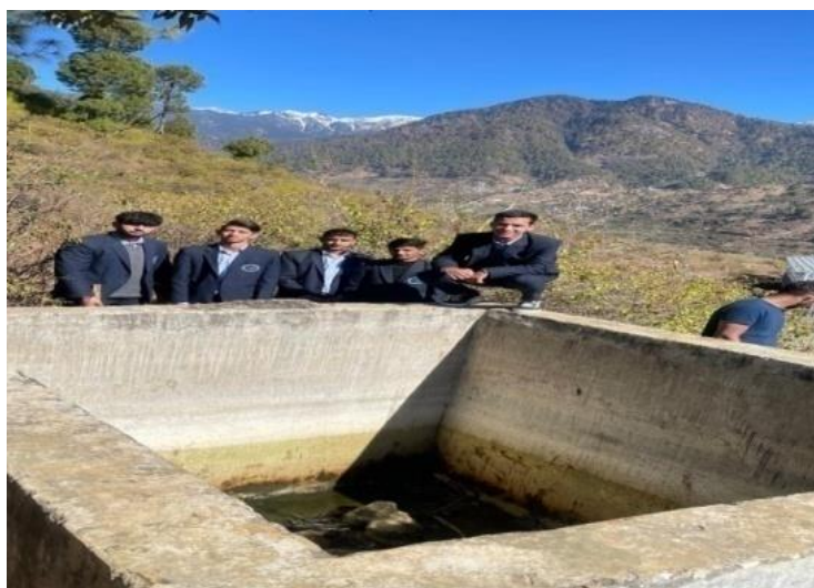
Fig 6.8: Cleaning of water tank (before cleaning)
