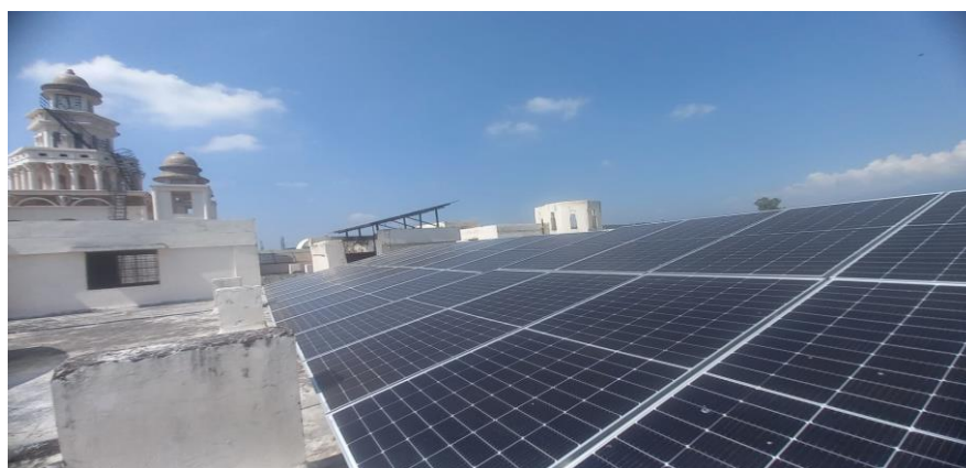
Fig. 1.7: Installation of rooftop solar power plant
